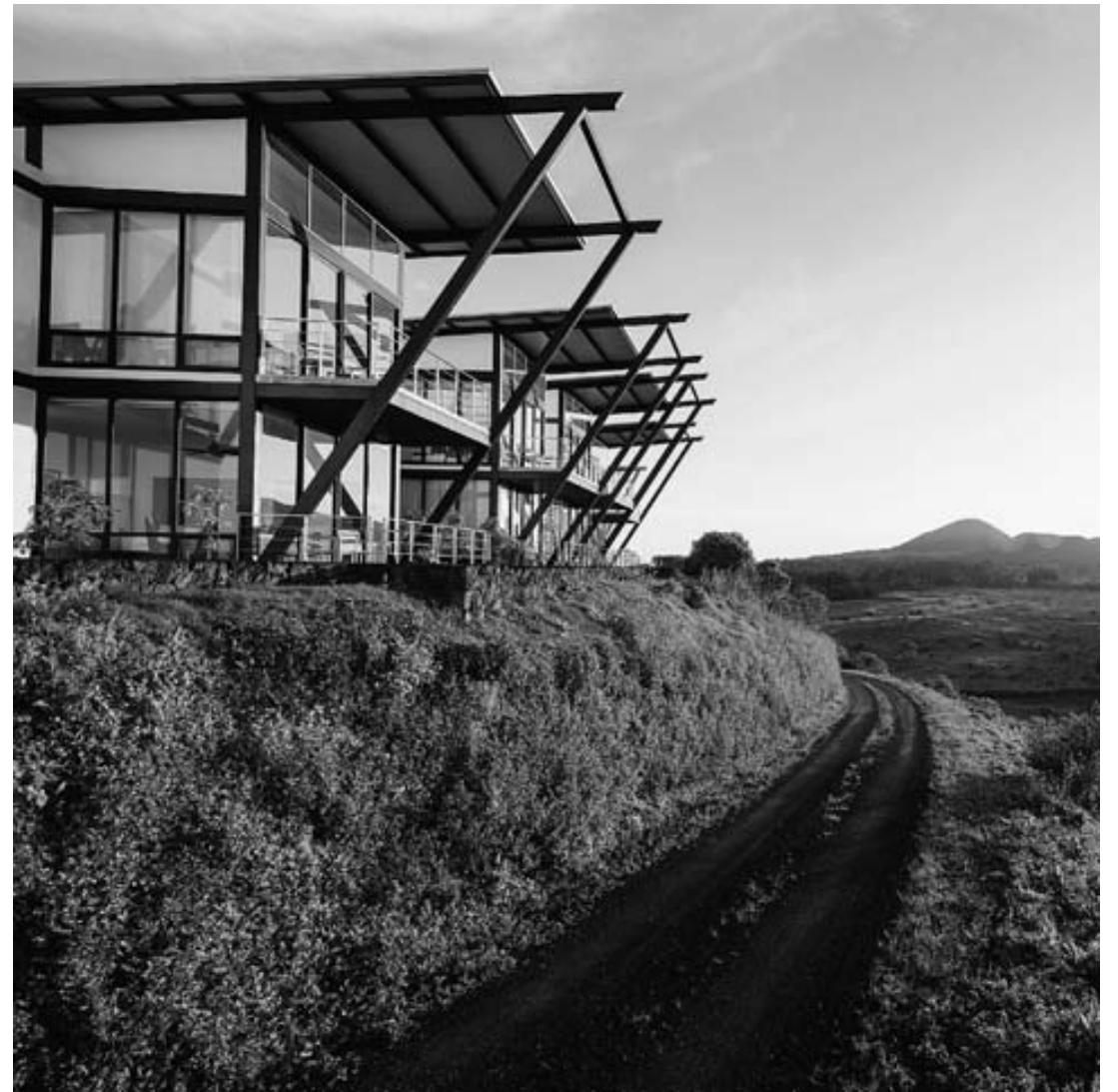
The Pikaia Lodge has 14 suites and is constructed of recycled steel, glass and natural stone.
